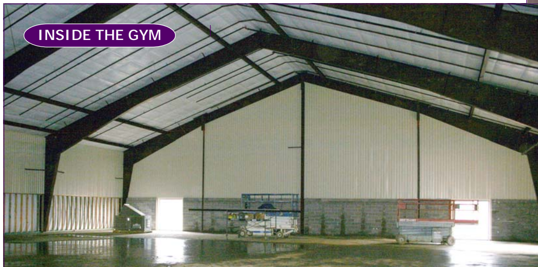
Gym walls and the roof are up; the floor will be wood. Locker rooms and a coach's office are being completed.
