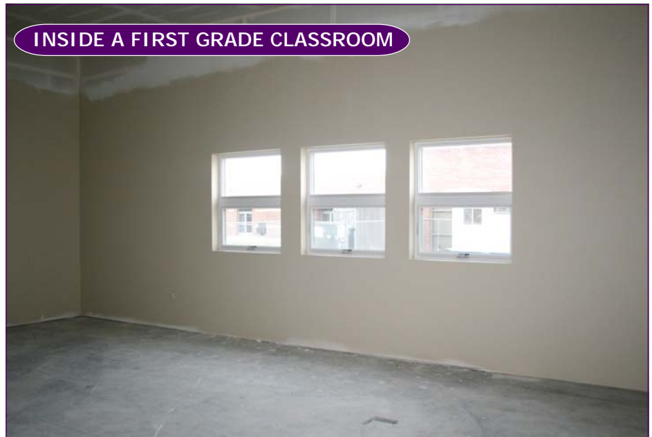
Classrooms on the east wing (two each of preschool, kindergarten, first and second plus alphabetic phonics), have been painted and will have ceilings hung soon. Classrooms on the west wing (two each of grades 6-8, plus a science room and art room) are ready to be painted. Classrooms on the north wing (two each of grades 3-5) are being framed.
