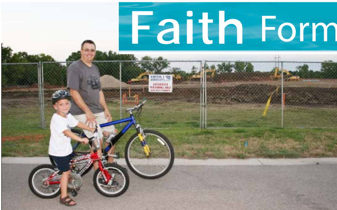
Brant Miller and his son Tyler, who will be in kindergarten, rode bikes over to check on the school construction progress this past week. View progress online at http://stmaryderbyrosehill.blogspot.com/
